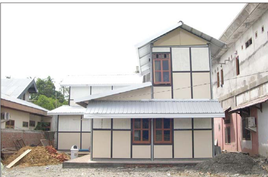
JRS teams in Aceh have utilized a unique model of replacement homes with a design from a Jesuit technological school in Indonesia. These structures minimize the use of wood which is scarce in northern Aceh. The hundreds of homes built by JRS are designed to be earthquake resistant and to last more than 40 years.
